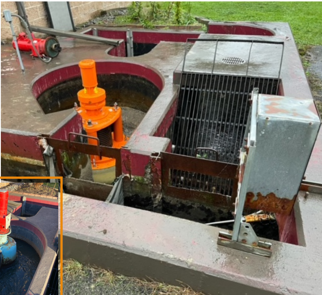
Retrofitting Chicago Pump 25M
