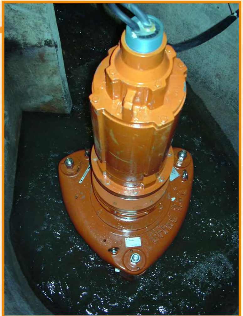
Basin of previously installed Chicago Pump 25M
